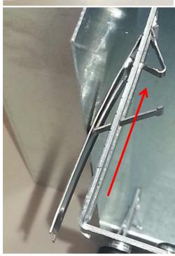
8. Once the spring clips pass through the neck to the wider section of the plenum the springs will extend fully preventing the diffuser falling out.
