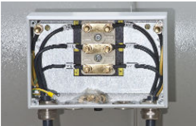
Fig. 22: Terminal box on the axial fan
